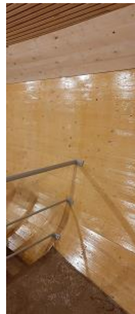
Wand strak in de lak
